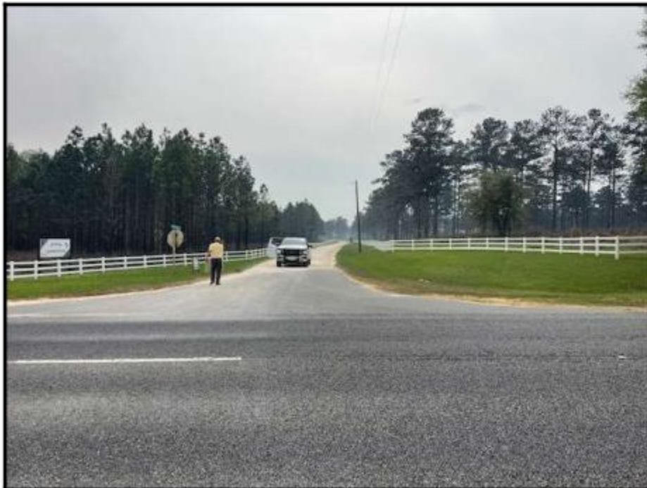
Photo 2: View of Avalon Rd as it extends S from E. Capps Hwy (subject right and left).
