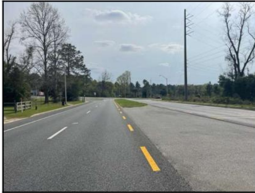
Photo 1: View of Hwy 19 as it extends S to E Capps Hwy; subject property at left in photo.
